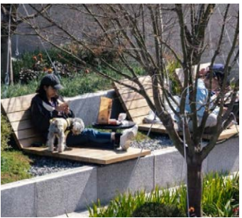
Timber Seat on Retaining Walls
