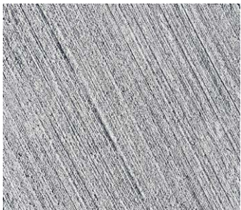
Concrete Paving Broom finish concrete
